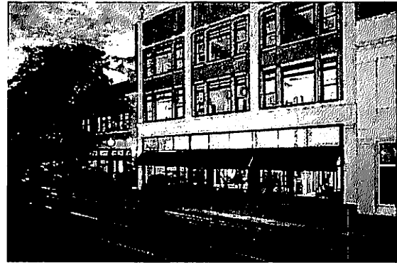
Corporate Headquarters, Sumter, SC
